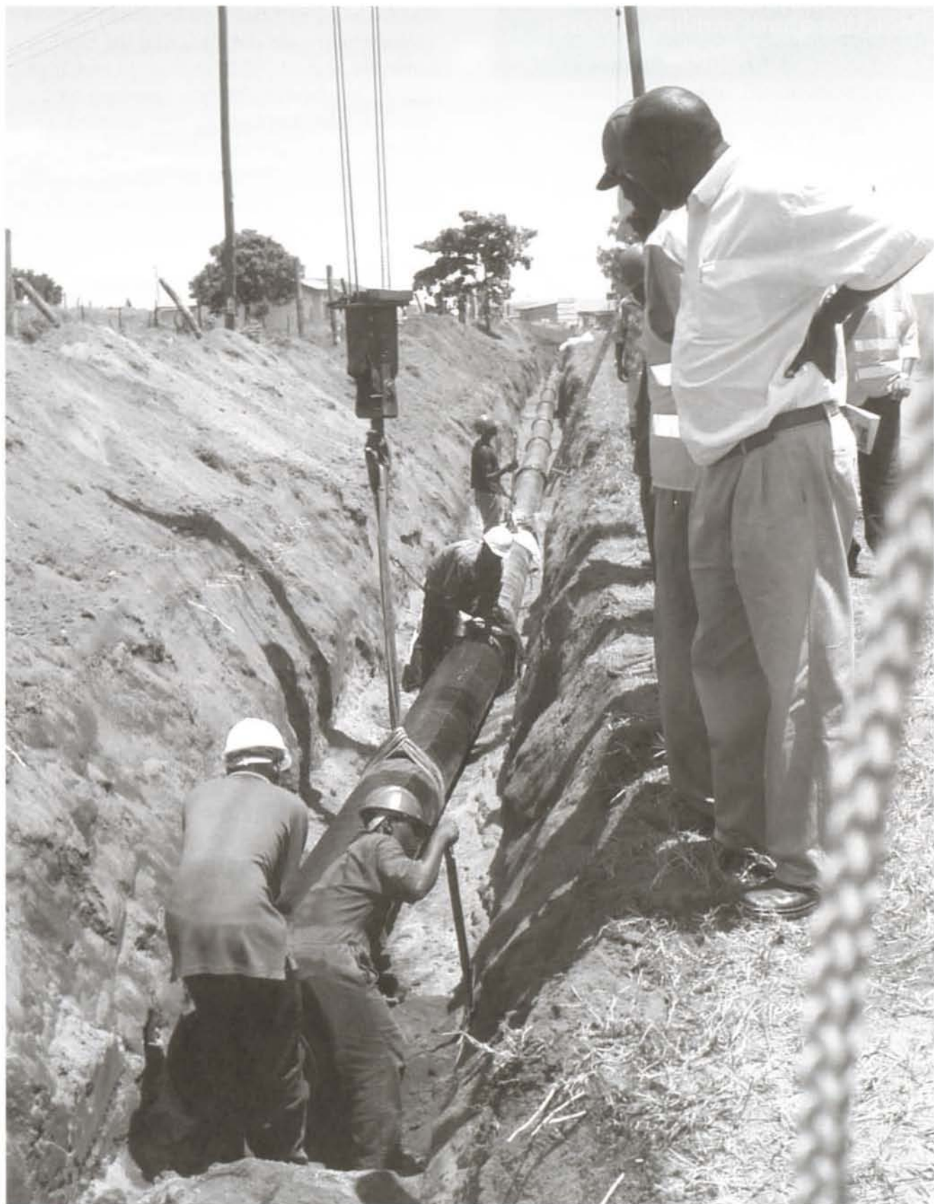
Laying of new pipes by NWSC
