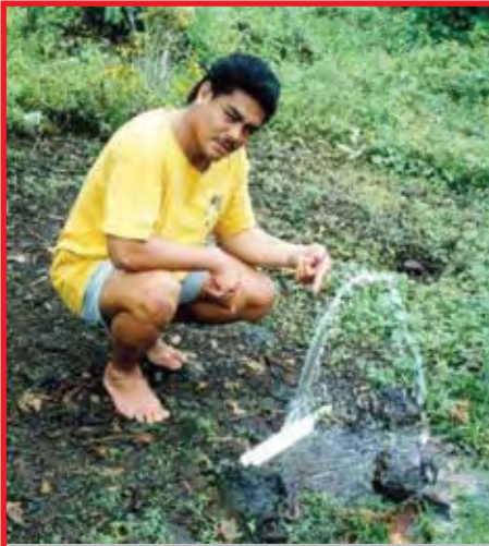
Typically more difficult to detect, service connection leaks result in significant water losses.
